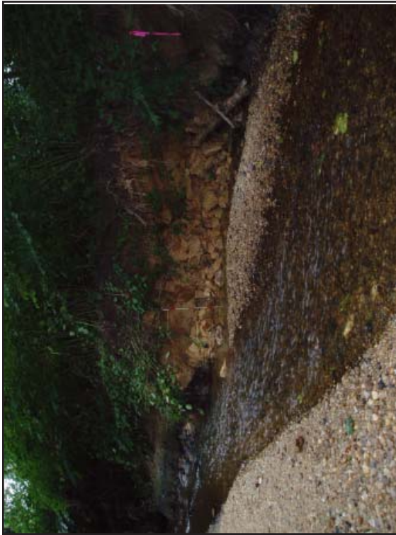
Figure 25: Location - Approx. 400 Feet Downstream of Powder Mill Road (Near X-1): Severe Streambank Erosion
