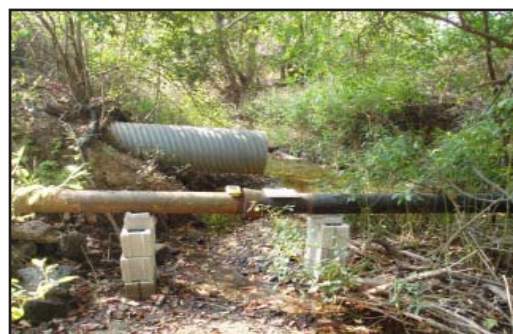
UBC-11 - Ductile Iron Utility Line Supported by Two Cinder Block Columns
