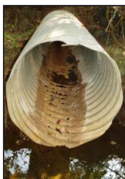
UBC-11 - 24 inch CMP stormdrain outfall
