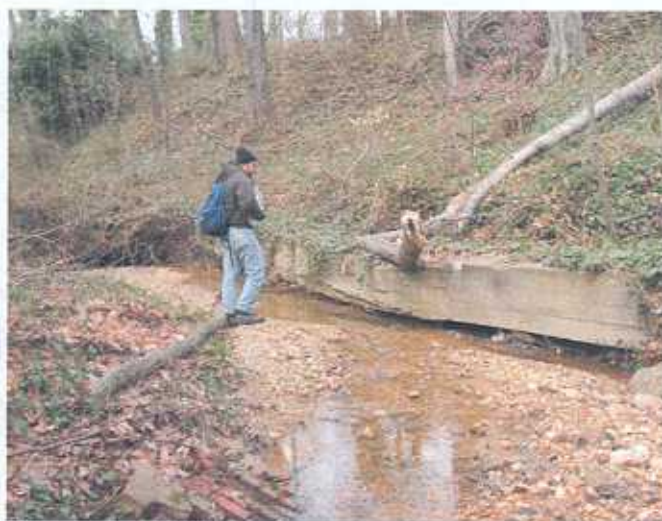
Figure 35 - Middle Reach - Existing Sewer Line and Concrete Encasement Condition
