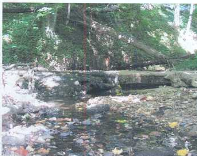
Figure 39 - Middle Reach - Complete Fish Blockage (X-19)
