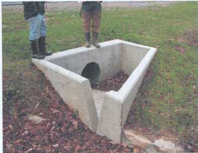
Figure 33 - Fort Davis Drive Storm Drain System - Flow Regulating Weir
