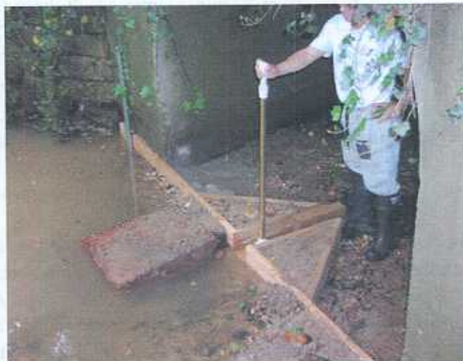
Figure 4 - Lower Reach 'A' - Four-Inch High Broadcrested Weir At Minnesota Avenue
