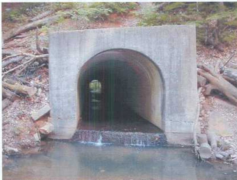
Figure 17 - Lower Reach 'B' - Complete Fish Barrier - 18.0-Inch Drop At Minnesota Avenue Culvert
