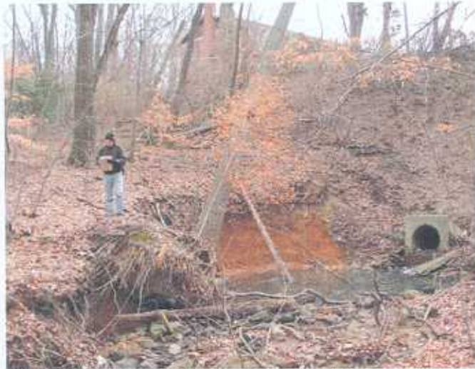
Figure 7 - Upper Reach 'B' - 33-Inch RCP Texas Avenue Storm Drain Outfall Area
