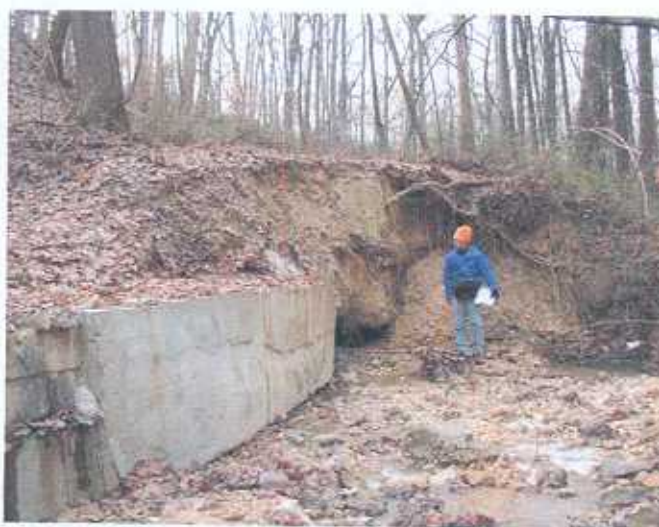
Figure 32 - Pope Branch - Upper Reach 'B' - Undercut Sewer Manhole
