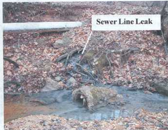
Figure 20 - Upper Reach 'A' - Sewer Line Leak Near 35 th Street (January 2001)
