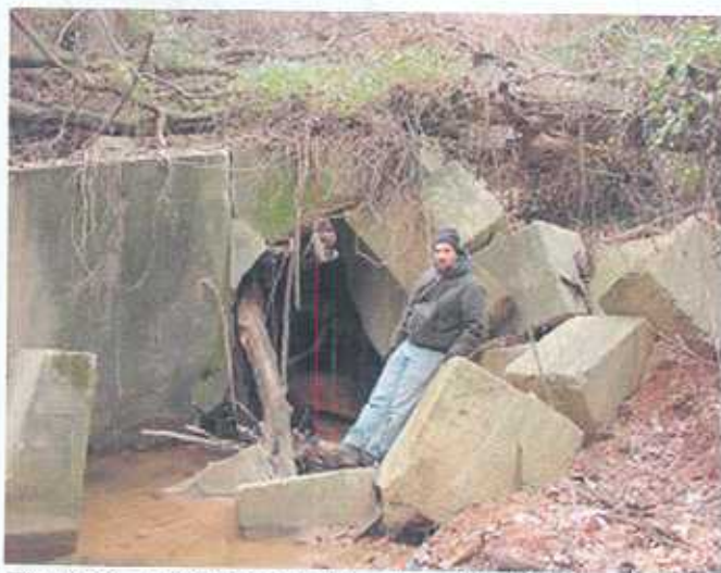
Figure 36 - Lower Reach 'B' - Complete Fish Barrier - Branch Avenue Culvert Endwall
