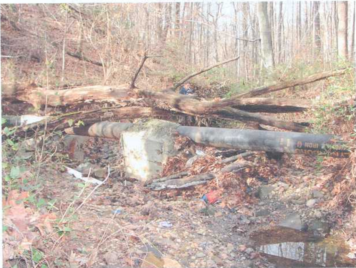
Figure 11 - Upper Reach 'B' - Undermined Sewer Line Support Pillars
